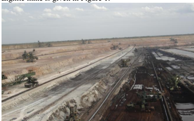
Figure 1 : view of lignite mine in operation
