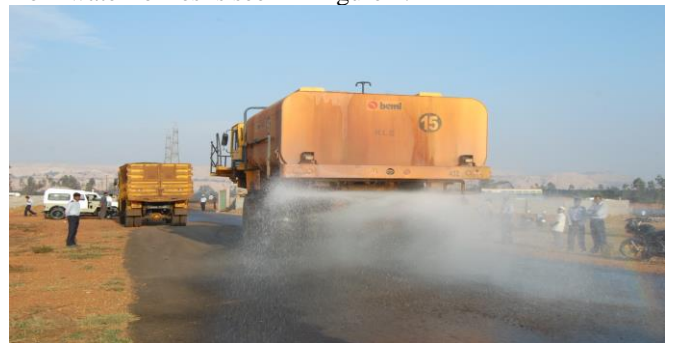
Figure 2 - Dust suppression on haul roads by water spraying from water lorries
