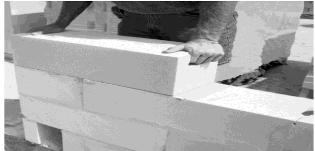
Fig.1. AAC block Masonry
