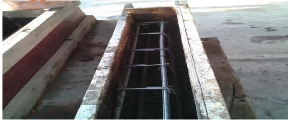
Formwork for beams
