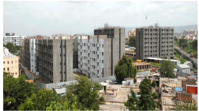
SLUM REHABILITATION PROJECT SITE
