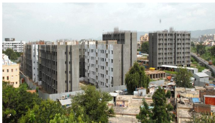
SLUM REHABILITATION PROJECT SITE
