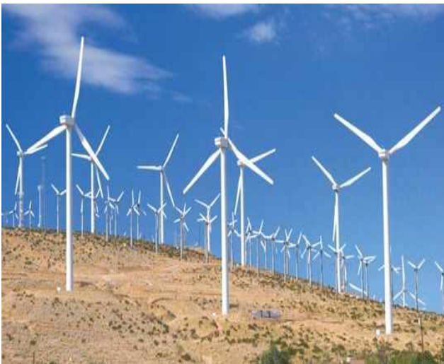
Fig. 8: Placement of Turbines
