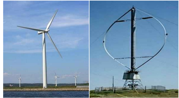
Fig. 2: Two basic wind turbines, horizontal axis and vertical axis
