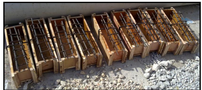
Figure (2): The moulds before casting of concrete
