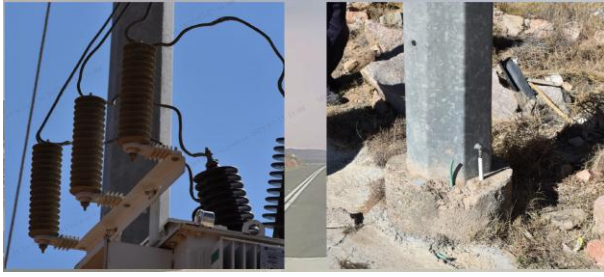
[Fig.3: Missing Ground Leads]
