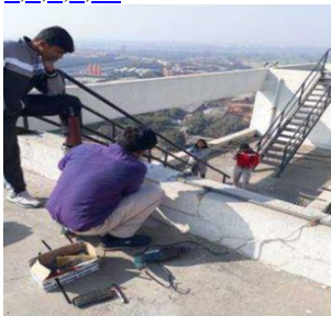
Figure 7 Antenna Installations at NIC-NKN
