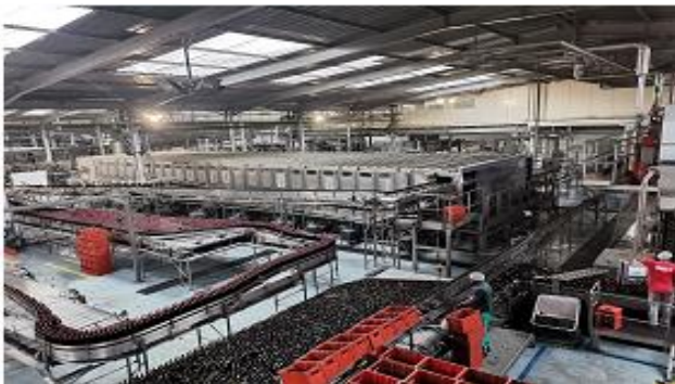
Fig. 2. Overview Image of The Equipment
