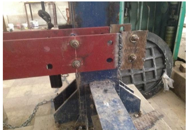
Fig. (7) Steel beam connected to the existing column
