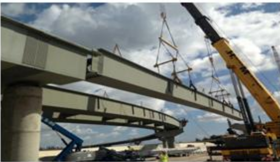
Fig. 1.Example of a Steel Plate Girders.
